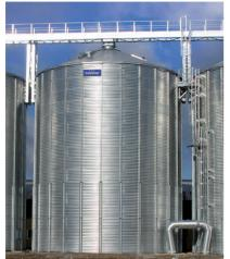
**STORAGE SILOS** Tornum storage silos are available with flat bottom or a 45° hopper in a wide range of sizes.
