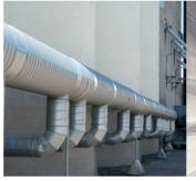
**KANALSYSTEM**<sup>™</sup> Dual function aeration/unloading systems for commercial installations. The Tornum Kanalsystem <sup>™</sup> can be used for any silo diameter or flat storage and will provide aeration with 100 % saturation and high unloading capacity, using only air.
